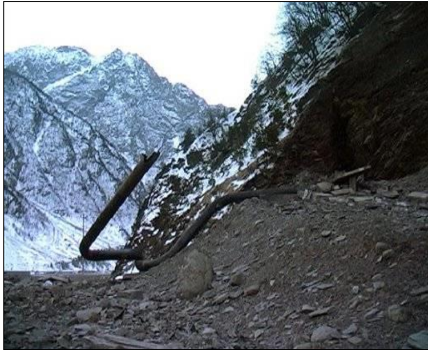
Exploded North-South pipeline 2006
